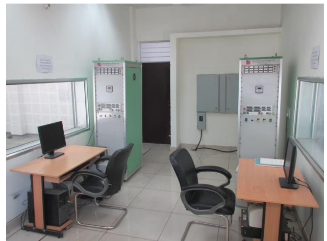
Dynamometer control room
